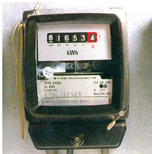
Figure 46. This is a domestic electricity meter. The reading in this meter shows the number of kilowatt-hours (or units) that have been used. The reading from this electricity meter is used to prepare our monthly electricity bill.
