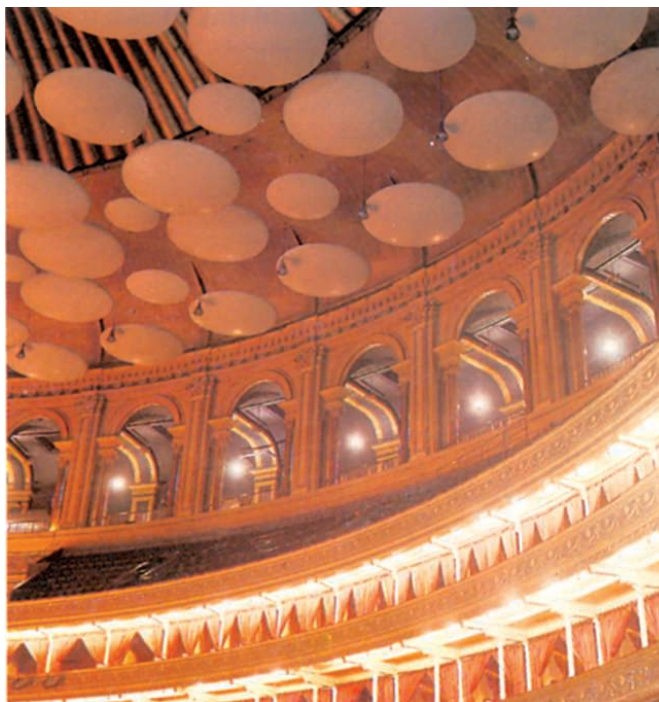
Figure 43. The 'mushroom' like panels on the ceiling of this Concert Hall are sound absorbers to reduce the reverberations (unwanted echoes).
