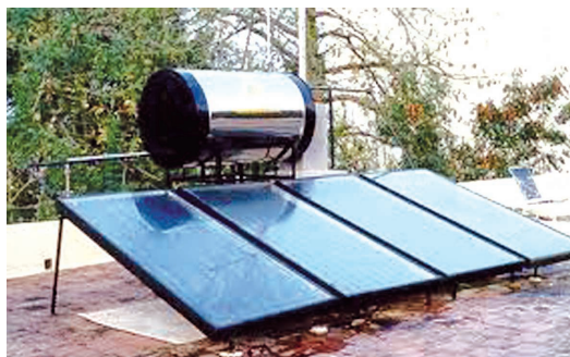
Figure 62. Solar water heater.
