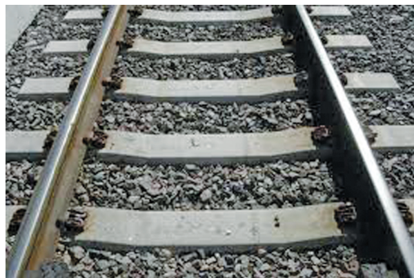
Figure 50. Concrete sleepers (or wooden sleepers) are kept below the iron rails of railway track so that the weight of passing train is spread over a large area of ground and the track may not sink into the ground.
