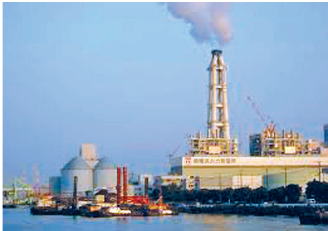
Figure 52. This is a thermal power house (or thermal power station). At a thermal power house, coal (or natural gas) is burnt to obtain heat which then boils water to form steam. The high pressure steam turns the steam turbines. The steam turbines then drive generators (or alternators) to produce electricity.
